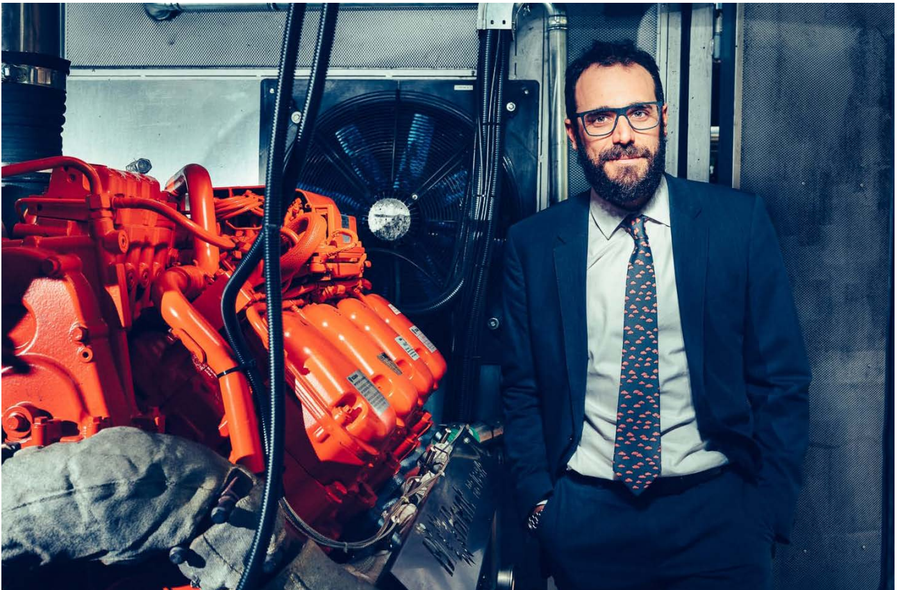
Mario Carraro of Mecc Alte says the company has been achieving fuel savings of 10 percent by using cogenerators from BioBrent powered by Scania.
